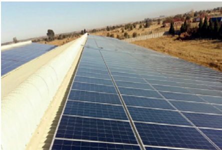
Rooftop structure with PowAR Snap® - SOUTH AFRICA
